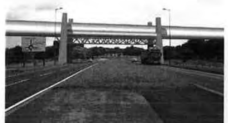
Image 3-4 Conveyor crossing the A1085 road (looking from Lord McGowan Bridge): 'truss' option
