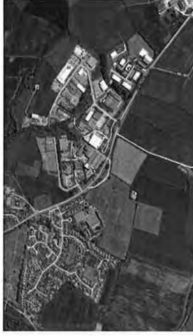
Figure 7.1 Broad Extent of land required for the Construction Village and Park & Ride
