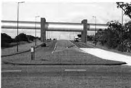
Image 3-1 Conveyor crossing the A1085 road (looking towards Lord McGowan Bridge): 'simple' option
