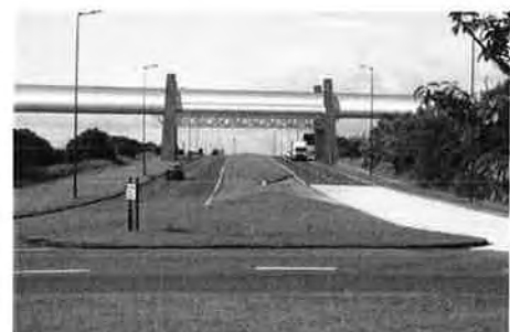
Image 3-3 Conveyor crossing the A1085 road (looking towards Lord McGowan Bridge): 'truss' option
